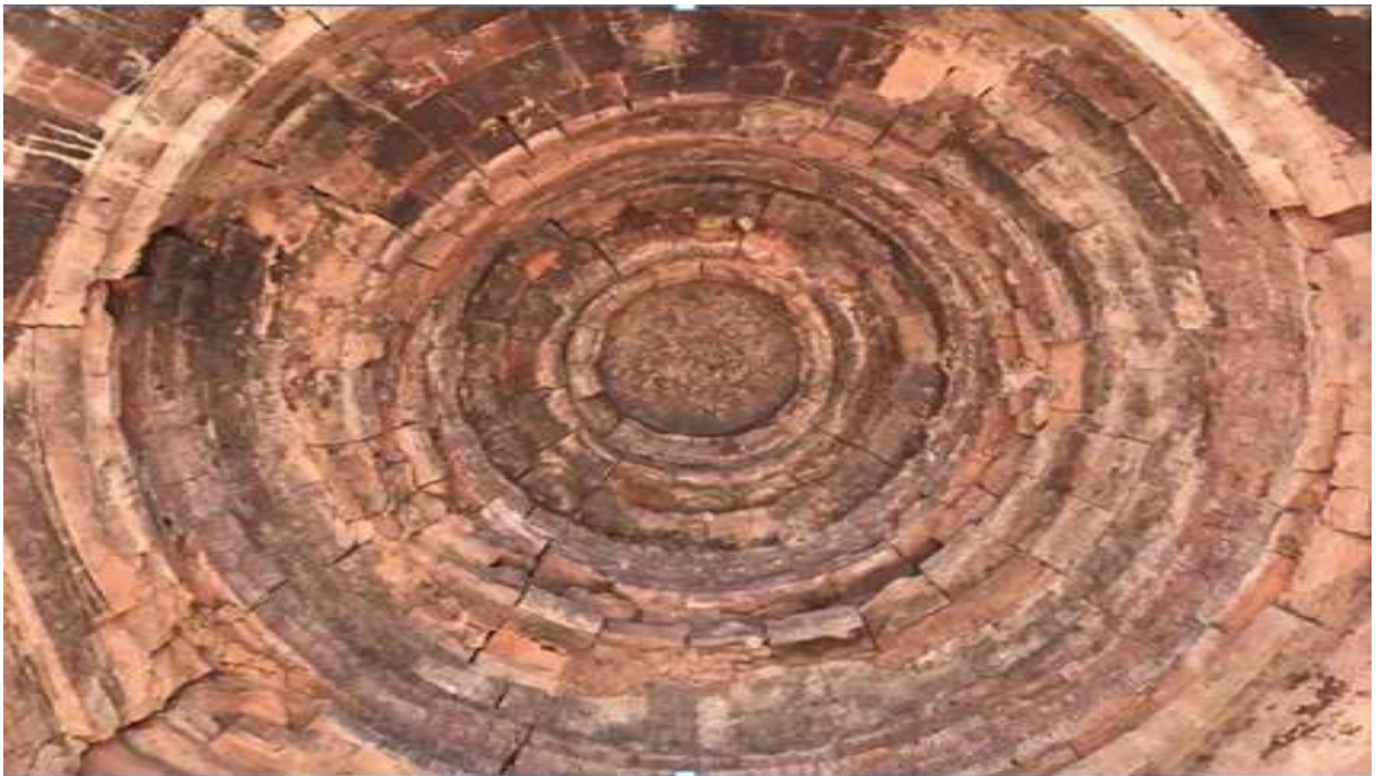
Fig14. Interior view of the dome showing concentric rings of bricks
