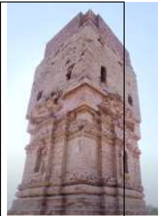
Fig.4. Pattan Munara that also might have served as lighthouse or watchtower at some time of its existence, while also serving as the temple.
