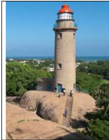
Fig.2. Mahabalipuram Lighthouse is located in Tamil Nadu, India. Courtesy: https://en.wikipedia.org/wiki/Mahabalipuram_Lighthouse# :
