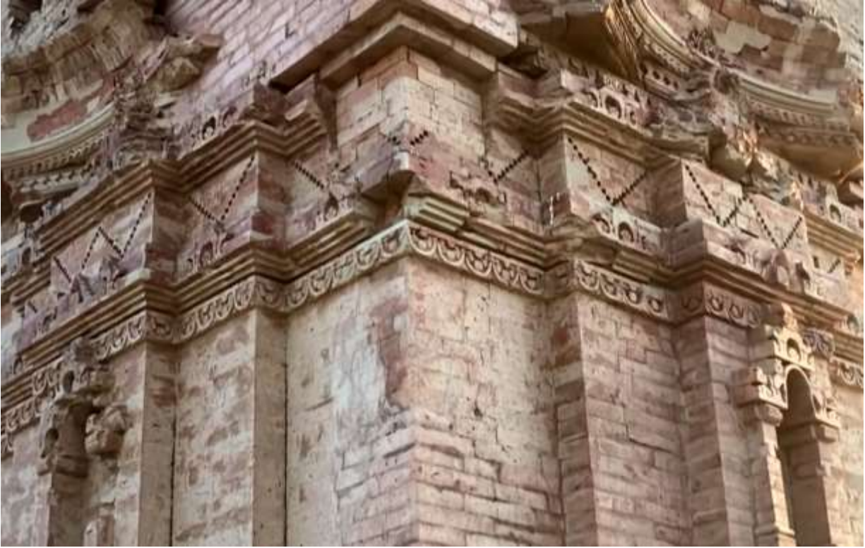
Fig.11. Arch-headed panels ornamented with a course of carved bricks visible.
