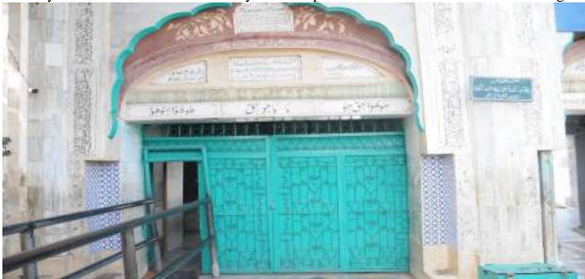
Picture 10: Outer view of the main gate to the complex
