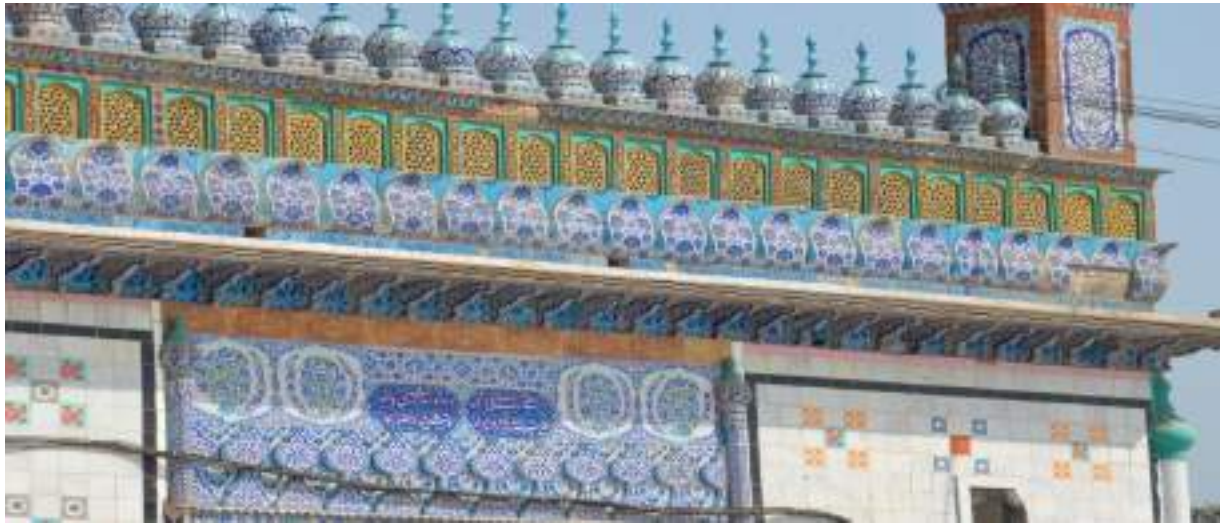
Picture 9: Blue tile work and lattice work on the parapets and frieze
