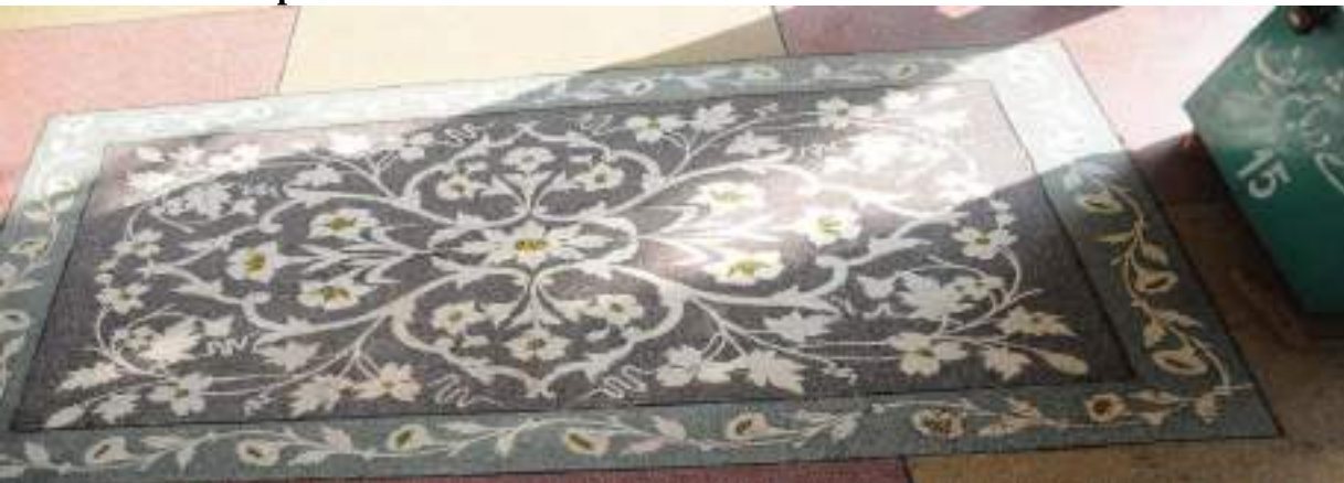
Picture 15: Veranda floor
