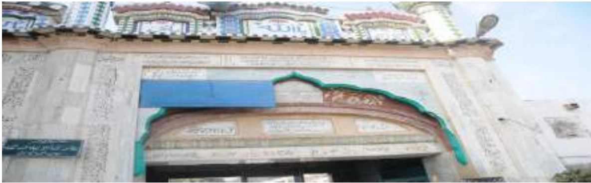
Plate 18: Front facade (darbar entrance)
